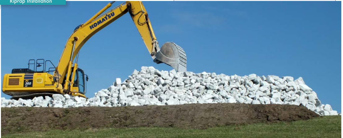
Riprap Installation
