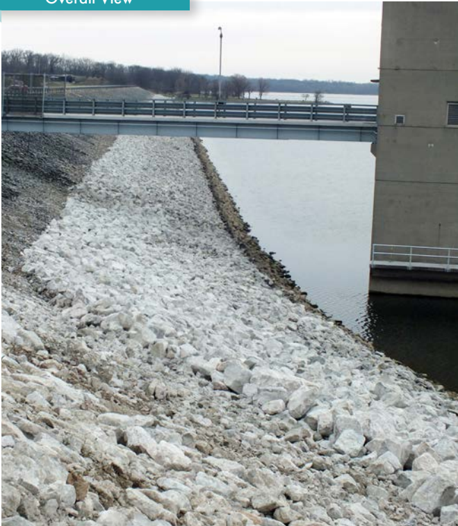
Riprap Installation
